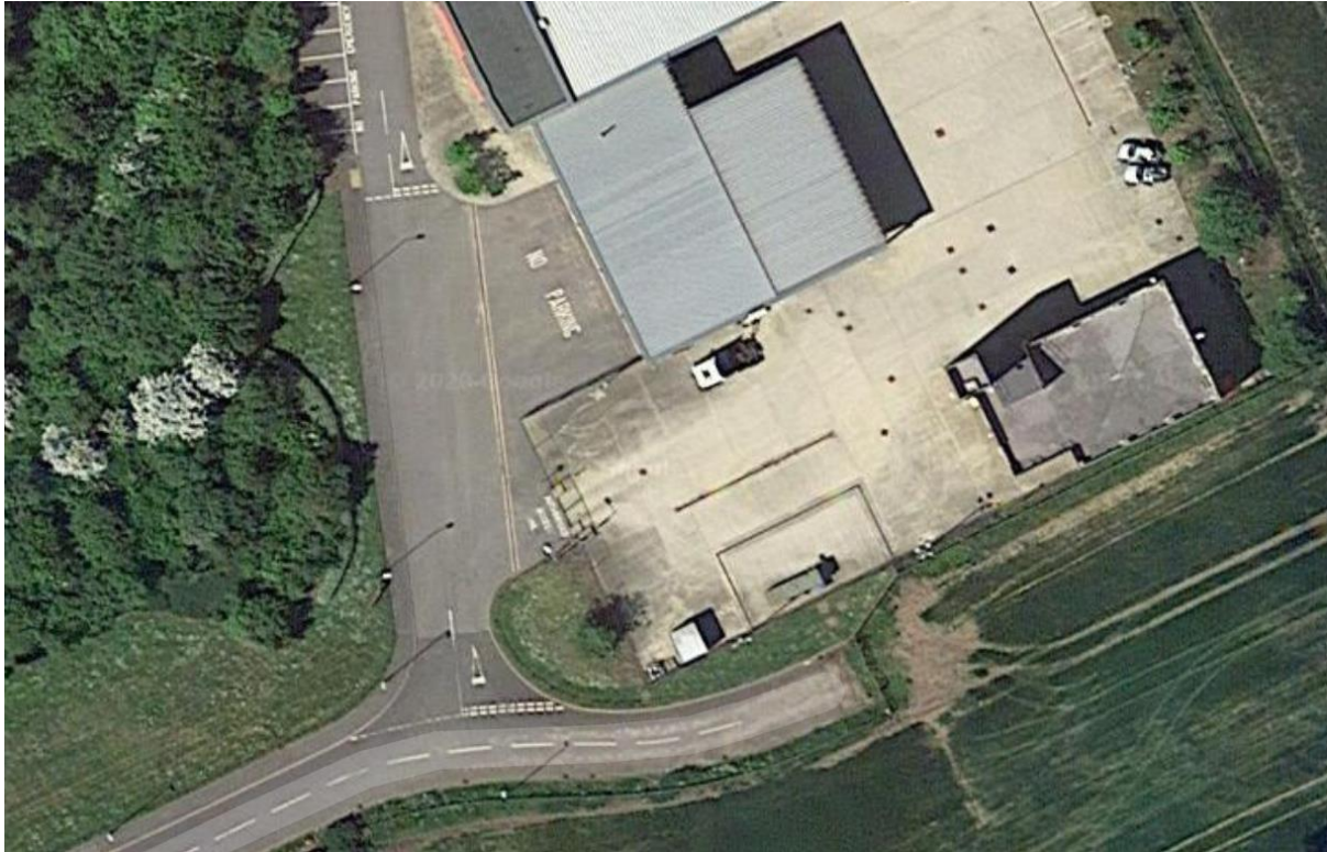
Fig 1. Aerial view of Bishop Auckland Fire Station and adjacent access road.
